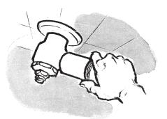
To mount angle stops on IPS stubs, especially on projects calling for large numbers of flush valves, eliminate wrenching by screwing a coupling and a short length of 1" pipe hand tight to the union outlet of the stop. Swing this "special tool" until stop is tight on stub. Job goes easier and faster. The chrome remains clean and unmarred.
